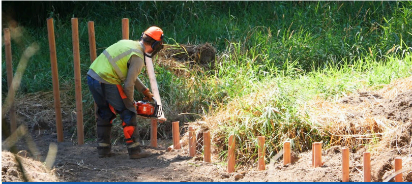
LCFEG Project Manager, Matt, uses a chainsaw to cut BDA posts to the proper height.
