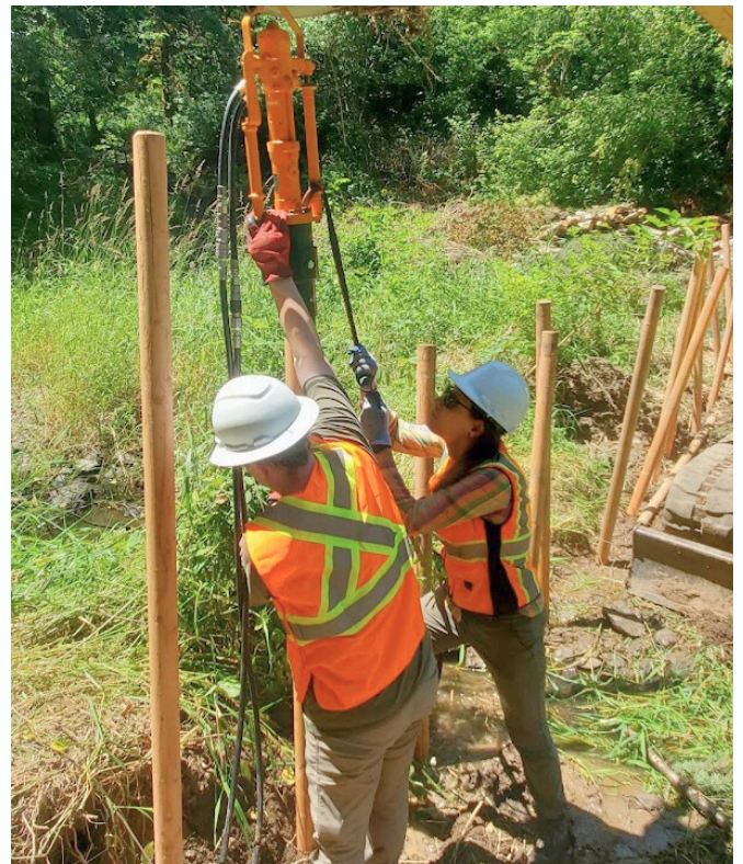
LCFEG Staff help to install BDA posts into the ground at Mason Creek.
